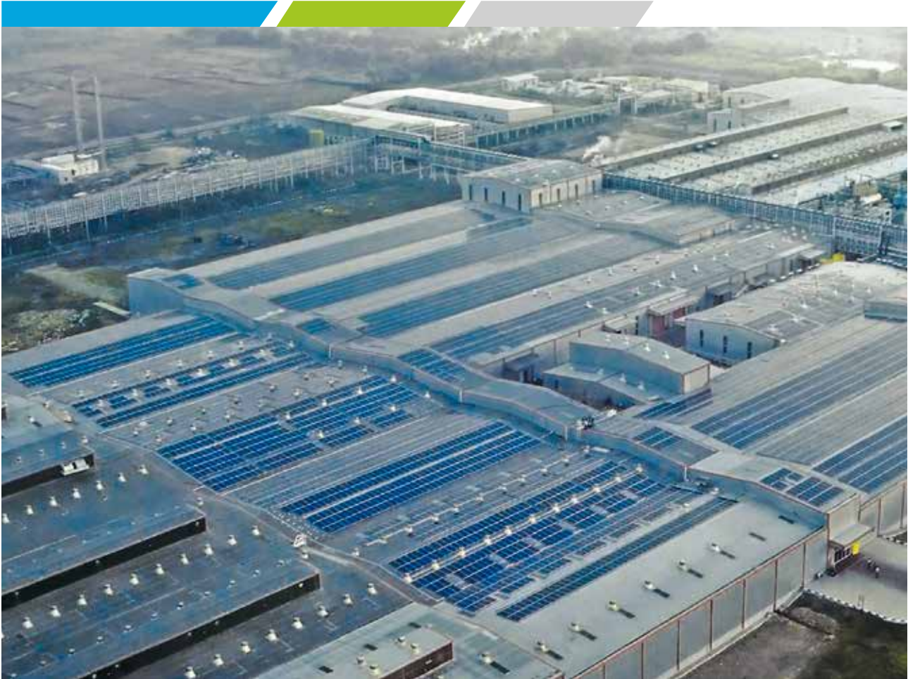
Aerial View of Roof Top Solar PV
