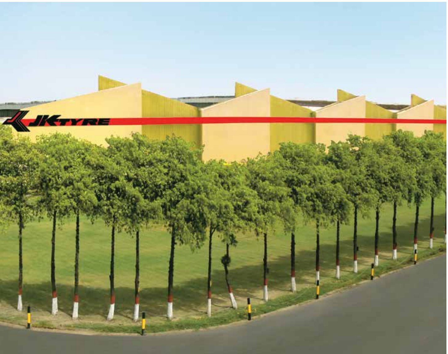
JK Tyre Plant, Banmore, Madhya Pradesh
